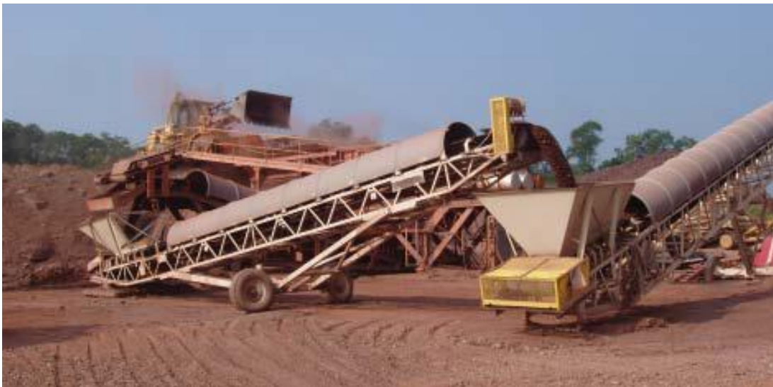
Figure (2.3): Clay or Shale being crushed and transported to storage area (Brick Industry Association TNT9, 2006).
